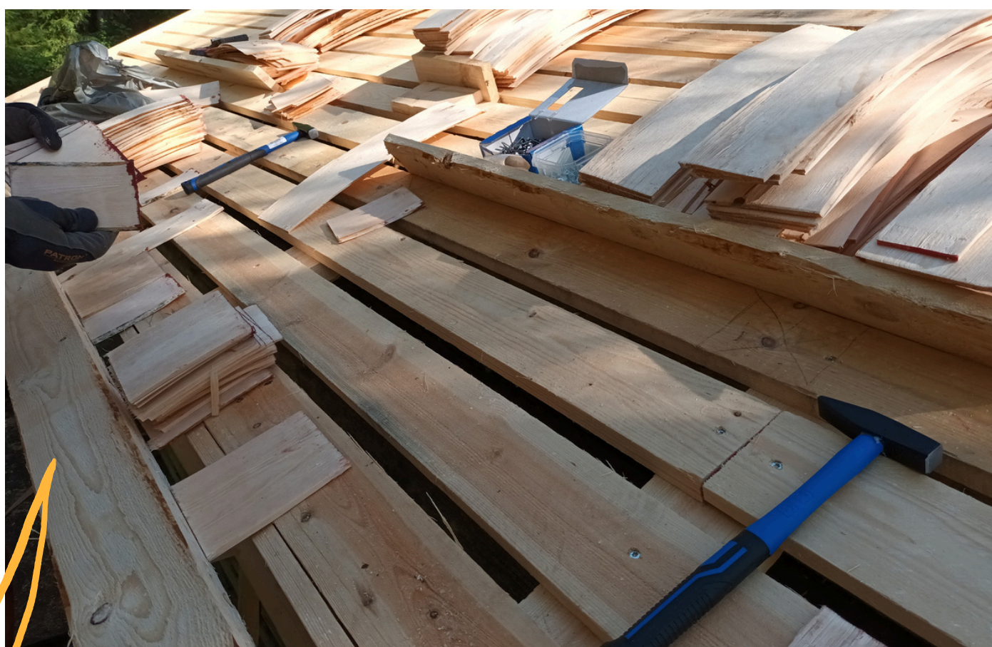
The first two layers have shorter shingles and they are nailed concave side up
