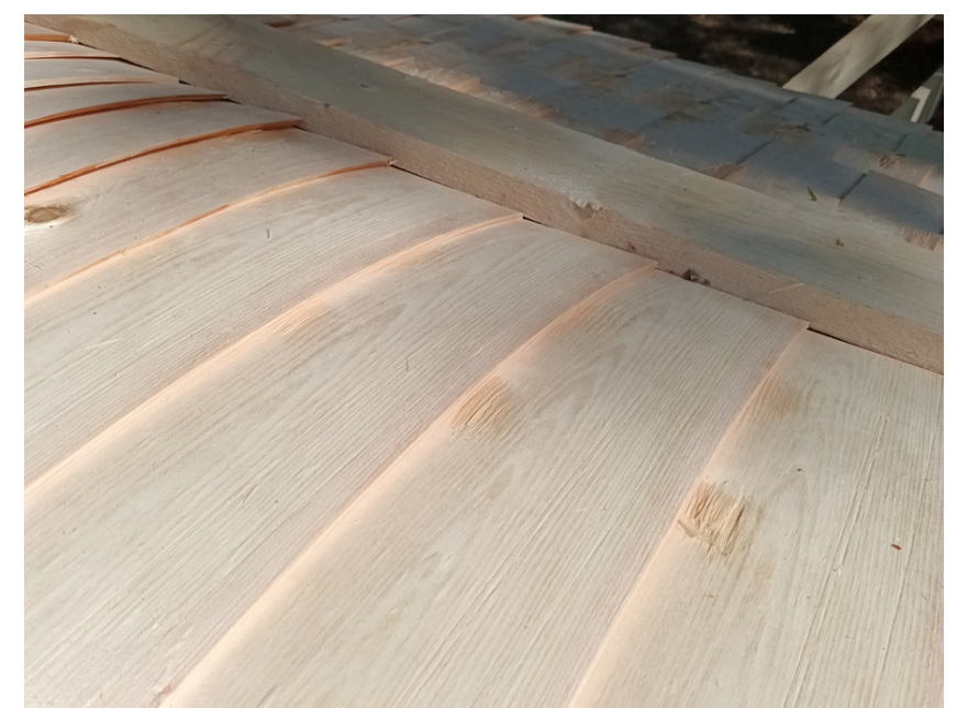
Shingles lined up overlapping
