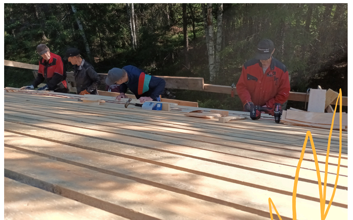
Building of the shingle roof
