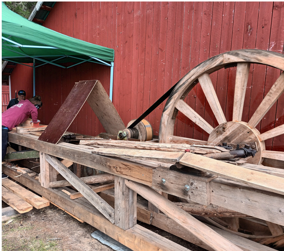
The plane for roof shingles in action
