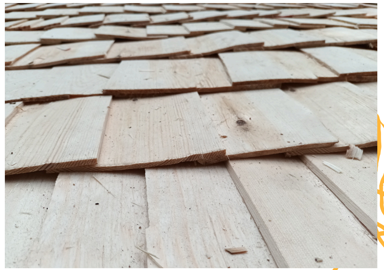
Completed shingle roof
