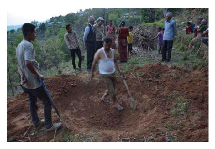
The diameter to depth ratio should be arround 2:1
